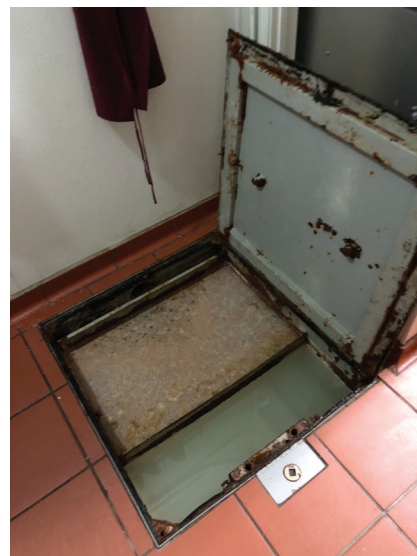
Example: Good condition, and working grease trap
