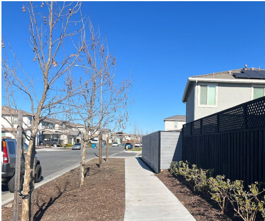
Figure 3: Unpermitted Extended Fence at 1381 Carriage Road (Photo is facing North on along the Westernly Property Line fronting North Gonzales Drive)
