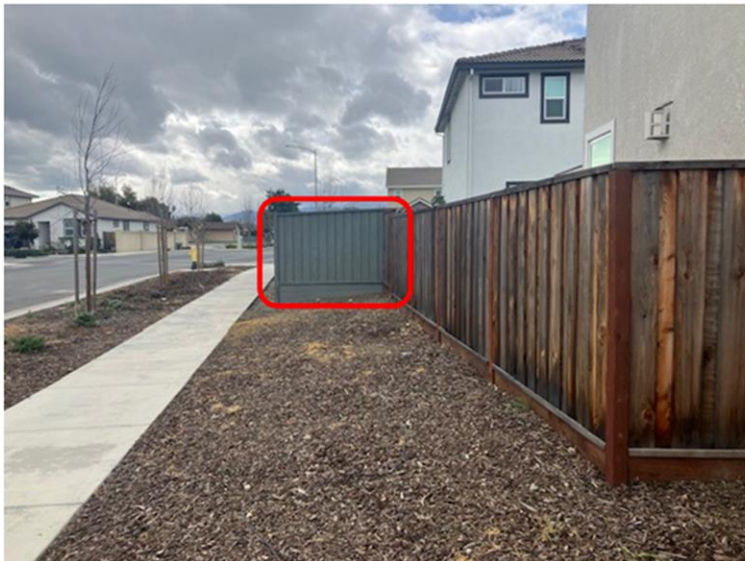
Unpermitted fence extension encroaching into the 10' utility easement.
