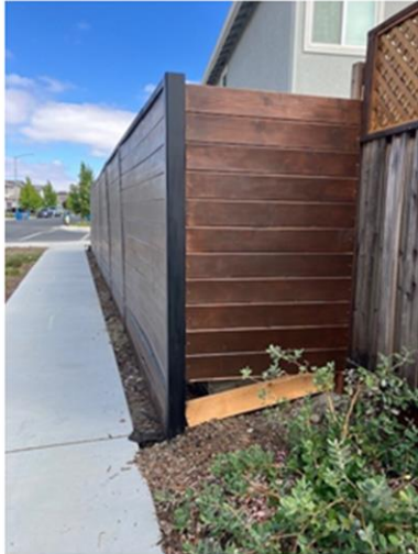
Rear extension of the fence line
