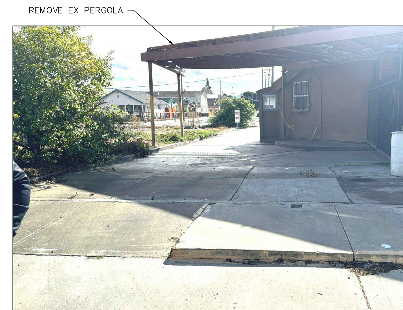
P2 - THE VIEW LOOKING SOUTH
